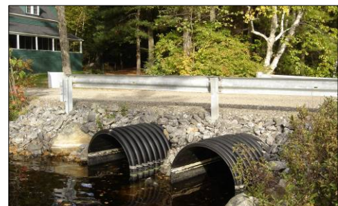
New culverts on Ramsdell Road
