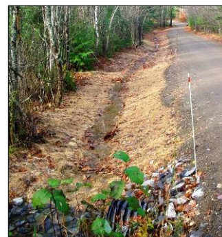
Casey Road – stabilized road surface and ditch
