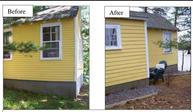
Camp Drive, West Bath – Property owner installed a dripline trench to infiltrate roof runoff and prevent soil erosion.
