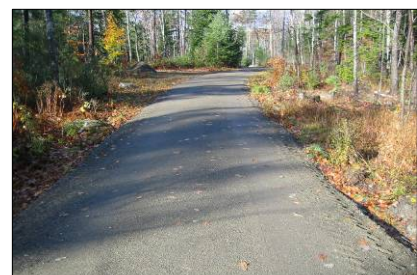
Pinney Road Project
