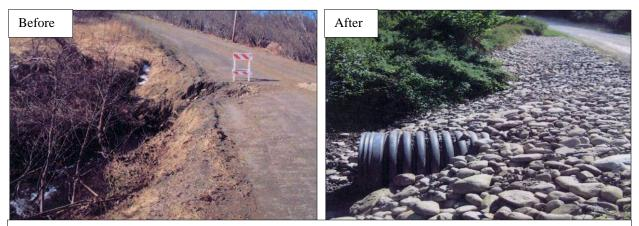
Severe erosion at Marden Hill Road stream crossing was stabilized by replacing the culvert, rebuilding the road, and armoring the culvert ends and ditches with riprap.
