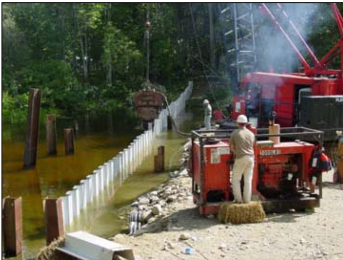
Construction workers building the roughened ramp
