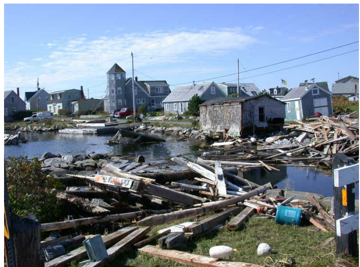
Figure 8: Storm damage at Prospect NS from Hurricane Juan in September 2003 (photo: Doug Mercer; from Leys 2009).
