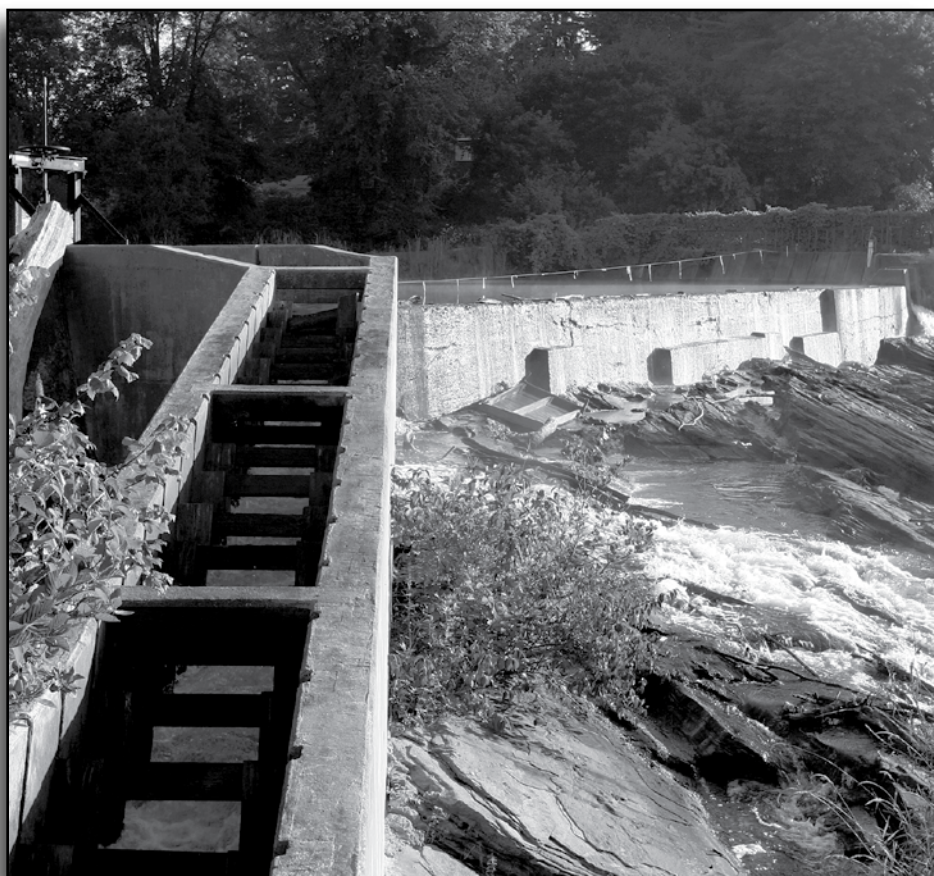
The Sparhawk Mill dam on the Royal River in Yarmouth, Maine, is a cement dam with a fish ladder. No water goes over the dam, and there is an eight-foot (2.4-meter) drop to rock ledge. Sediment has accumulated behind the dam. According to an inventory in 2005 commissioned by the state of Maine, the mill owner was still using the dam to generate power. At the time of the survey, debris had accumulated at the top entrance to the fish ladder, possibly interfering with passage of diadromous (sea-run) fish.
