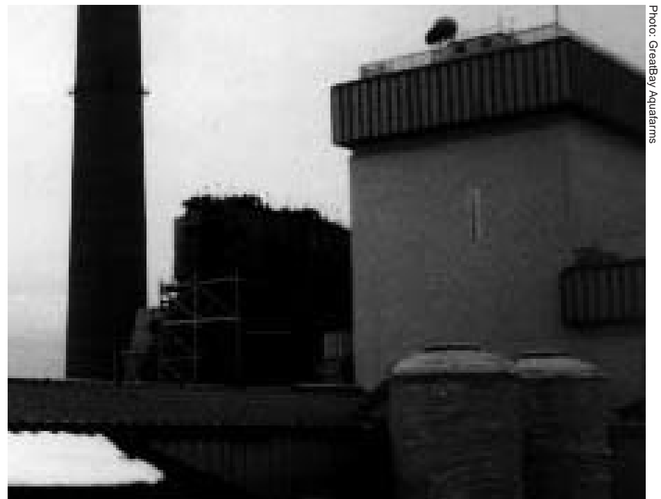
GreatBay Aquafarm's hatchery at a power station owned by PSNH/Northeast Utilities uses water tapped by the station and stored in two holding tanks (right).
