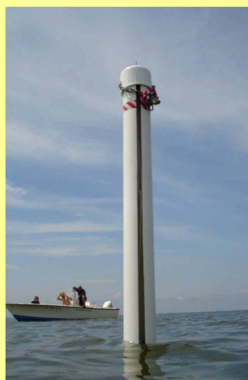
Continuous Sonde Installation
