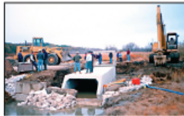
Crews install a culvert to restore water flows and fish passage to a tidal basin formerly blocked by a causeway.
