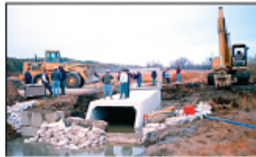
Crews install a culvert to restore water flows and fish passage to a tidal basin formerly blocked by a causeway.
